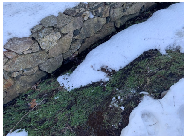
4 Brickyard Circle - 2 (Drainage Course)
