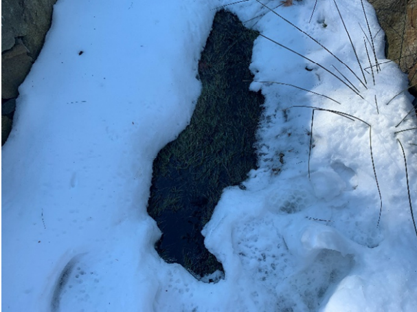
4 Brickyard Circle – 3 (Drainage Course)
