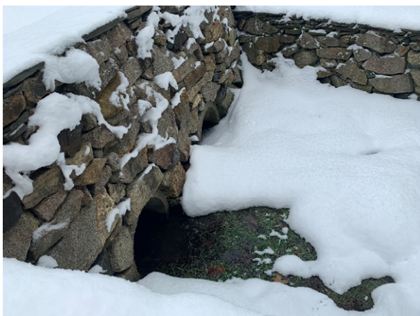
4 Brickyard Circle - 1 (Drainage Course)
