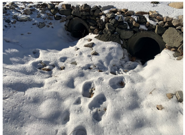
64 Gundalow - 2 (Drainage Course)
