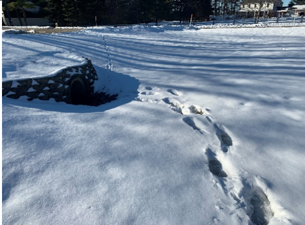
29 Gundalow - 1 (Drainage Area)
